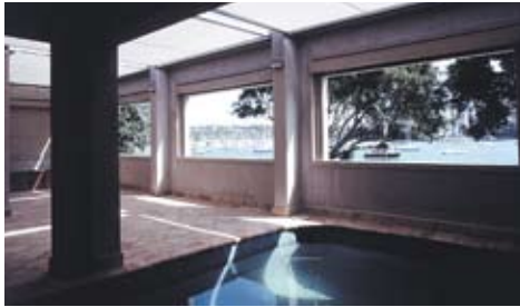
Air enters this building across the pool (thermal mass) via a semi-enclosed courtyard. It is evaporatively cooled before entering the building.
